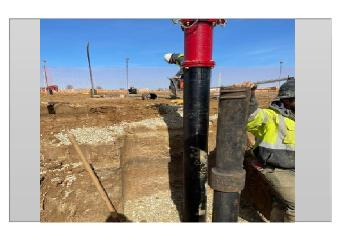
Hydrant and valve box installed off 6" DI line on far West side of site
