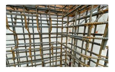
Lap pool wall rebar @ toe ledge
